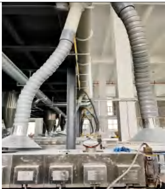
造粒废气集气罩
