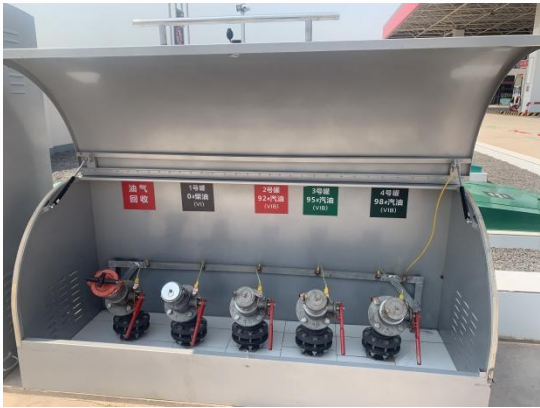
卸油口及卸油口油气回收
