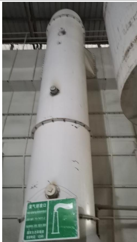
干燥机废气排气筒 (FQ-16217-2)
